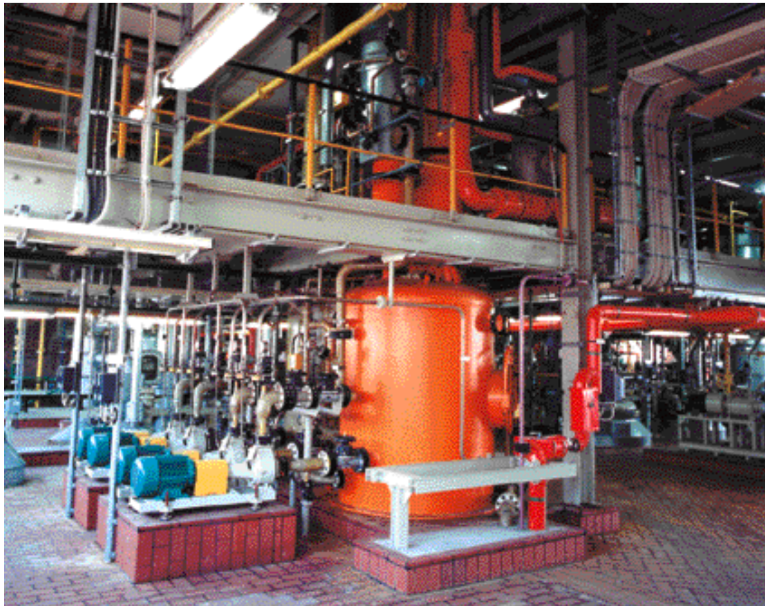
Example of a flue gas scrubber downstream of a exhaust gas and liquid oxidiser system
